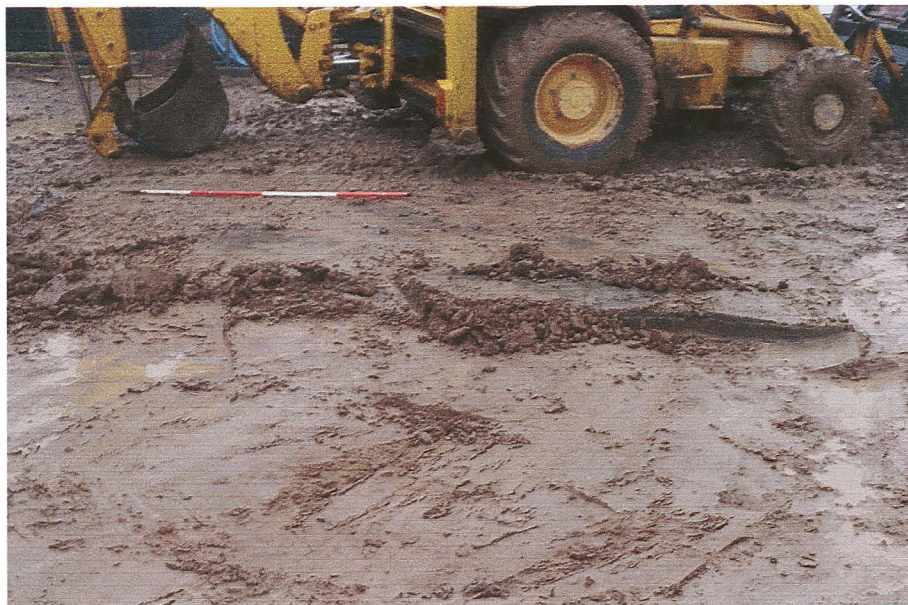
Fig.2 Wheel ruts looking west across the north of plot 10
