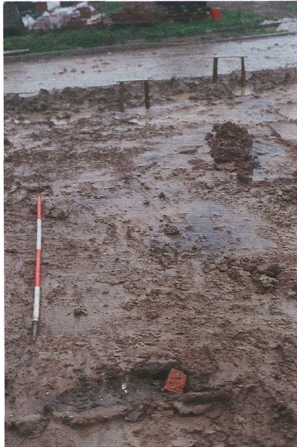
Fig.1 Wheel ruts looking north across plot 10 to the access road
