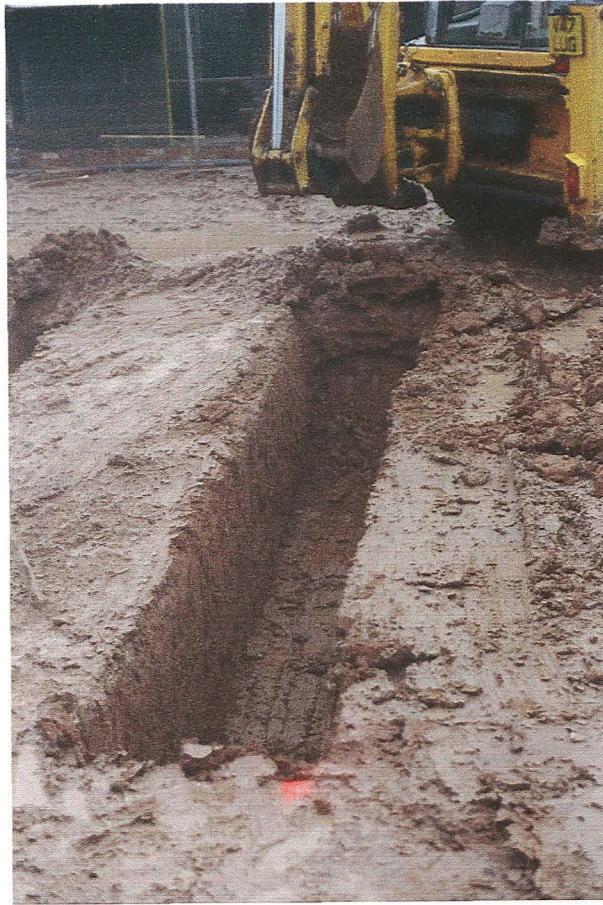
Fig. 3 Internal foundation trench looking west showing layer 101
