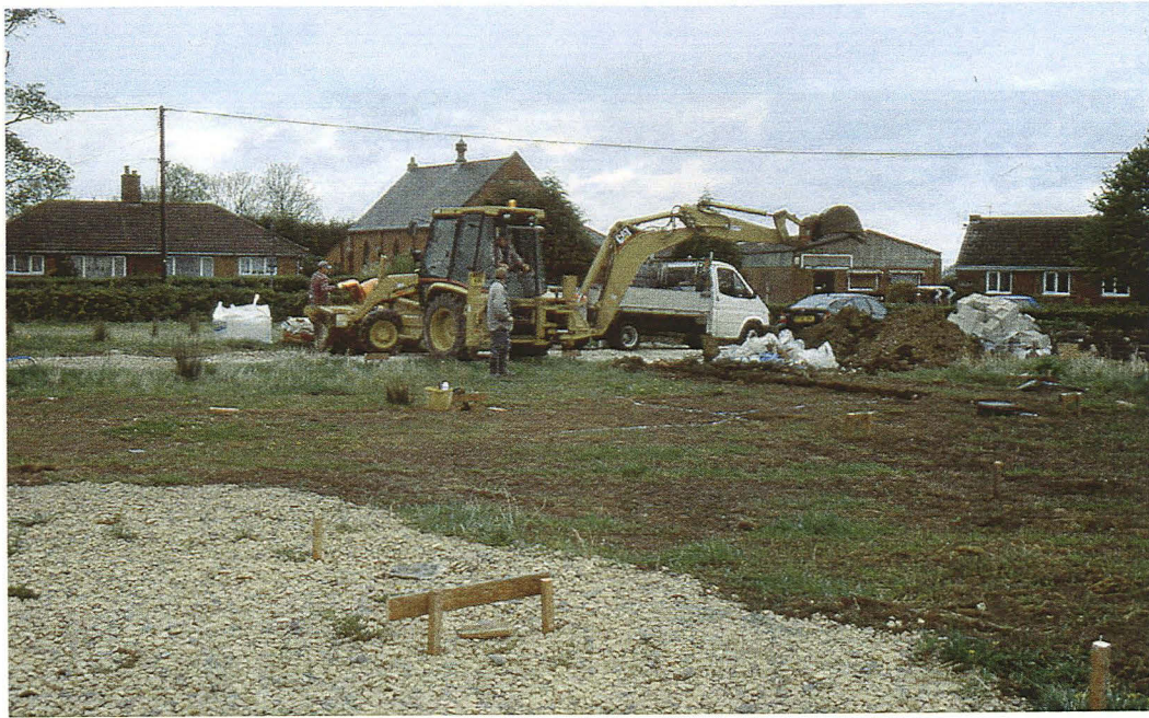
Plate 1 North facing view across Plot 4 prior to the commencement of machining.
