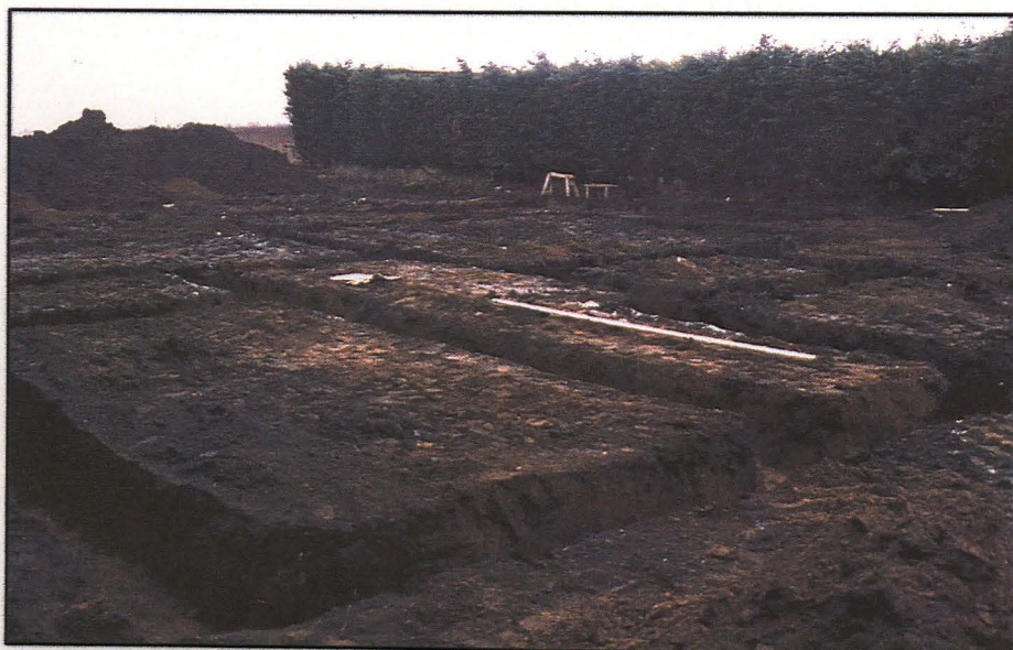
Plate 6 (left): the completed house plot foundation trenches, looking S.
