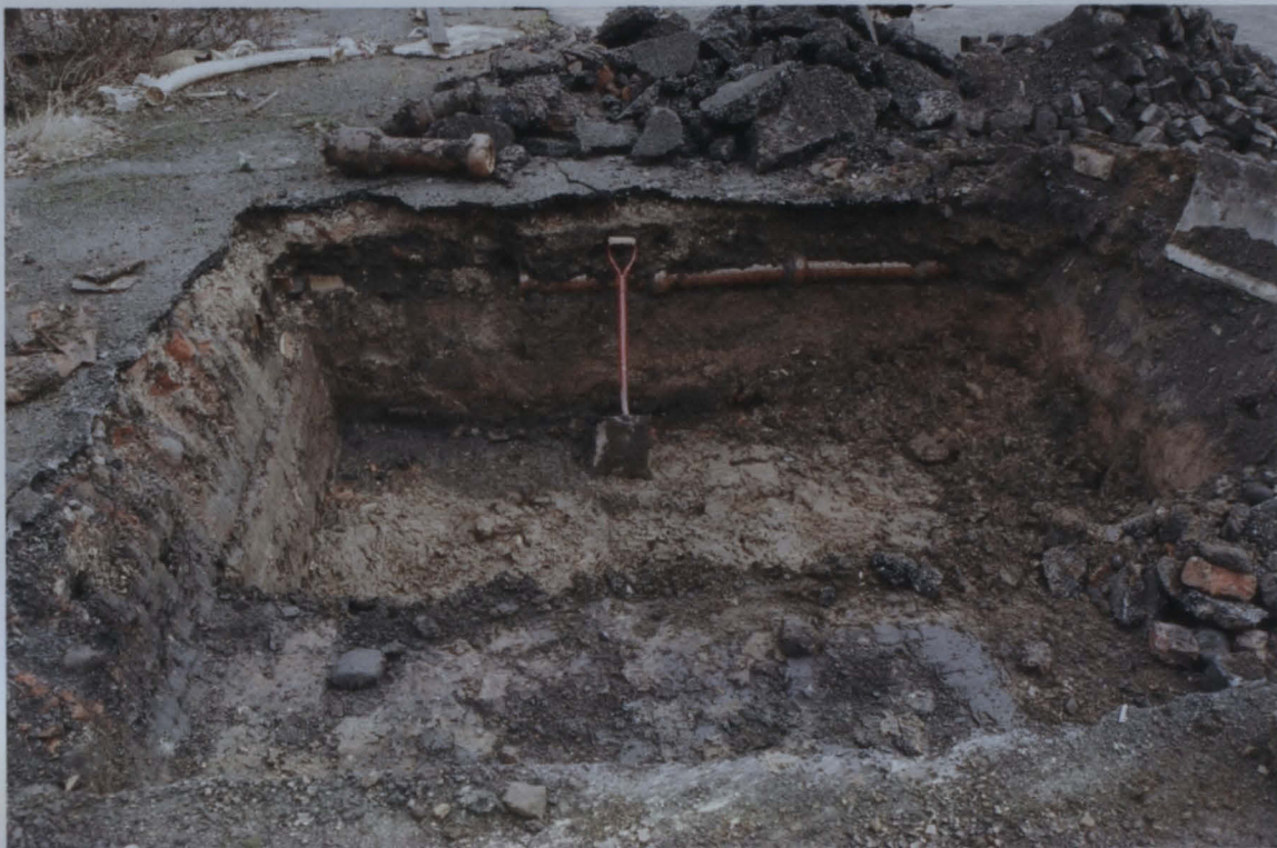
Pl. 5 Trench 2 during machine excavation showing services pipe 212, looking east
