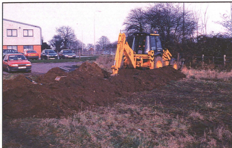
Plate 1 (above): Machining Trench 1, looking north-east.
