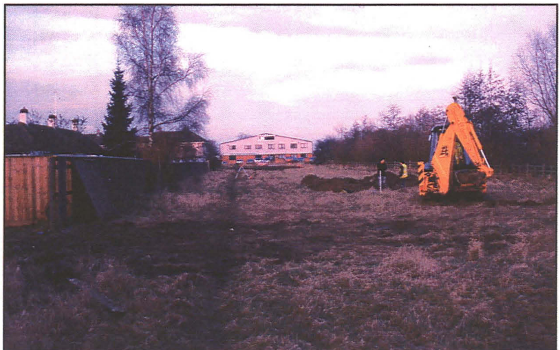
Plate 8 (below): General view of the site during backfilling, looking North.
