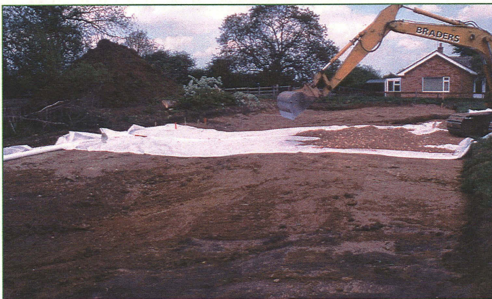
Plate 3: Laying geotextile and hardcore in the footprint of house plot 3, looking S.
