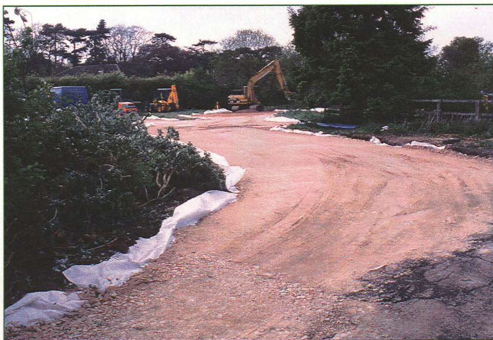
Plate 4: Hardcore and geotextile laid in the access road strip, looking NE towards house plot 3.
