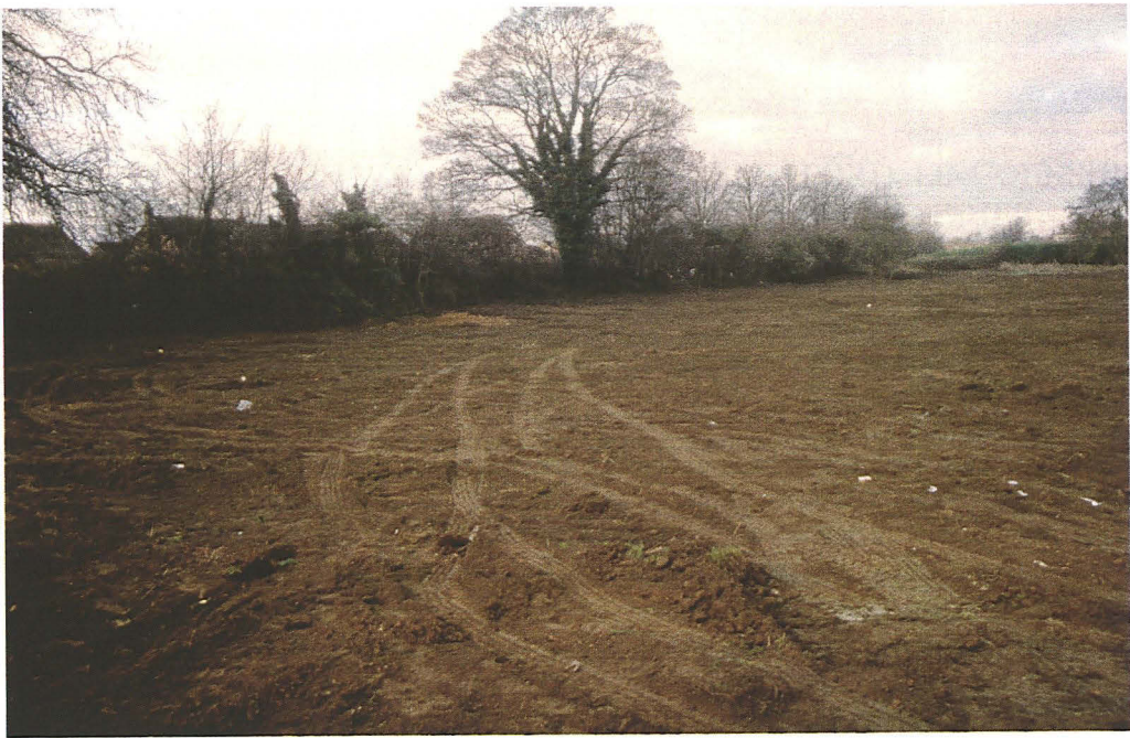
Plate 1 - General view across the development area, looking west
