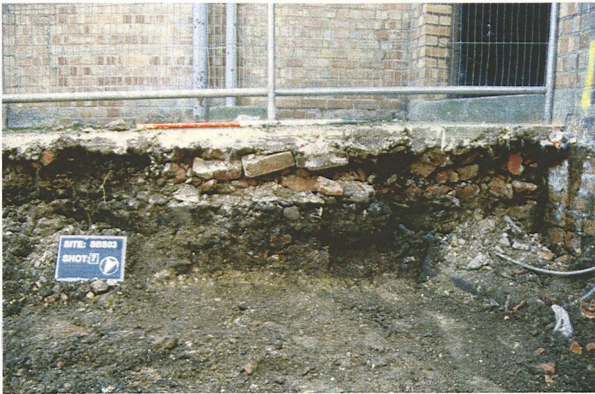
Plate 4 - Section 4 with the former topsoil (024) in the foreground, looking southeast
