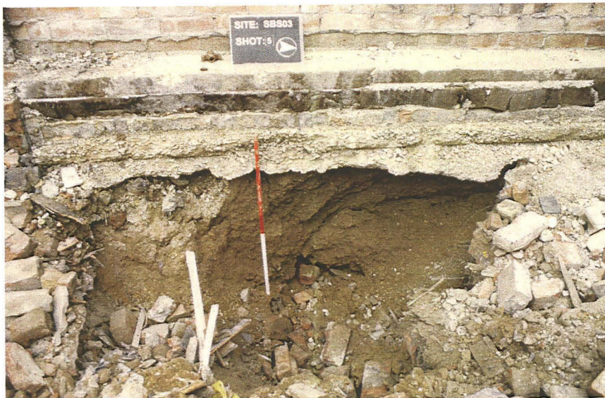
Plate 3 - Section 3 showing the infilled cellar, looking northwest
