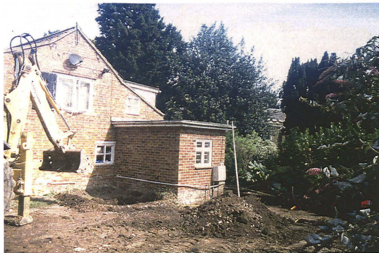
Plate 1 - General view of the development area with St. Edith's church in the background, looking northeast
