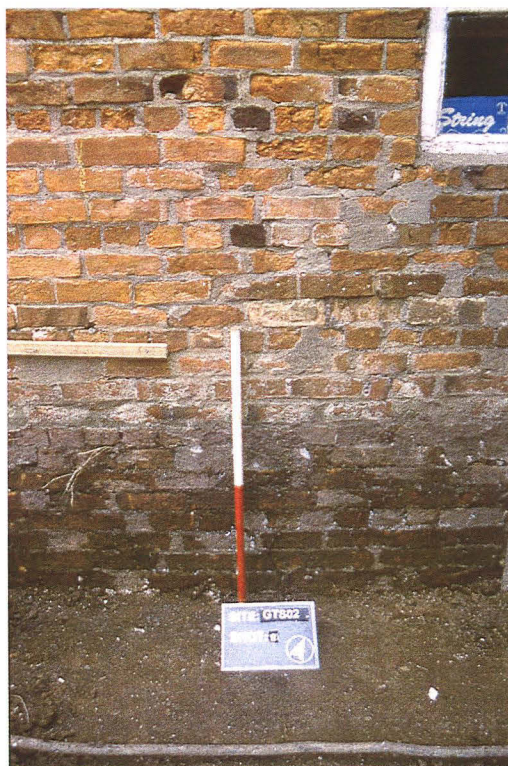
Plate 3 - Section 3 showing the extant wall (008), looking north
