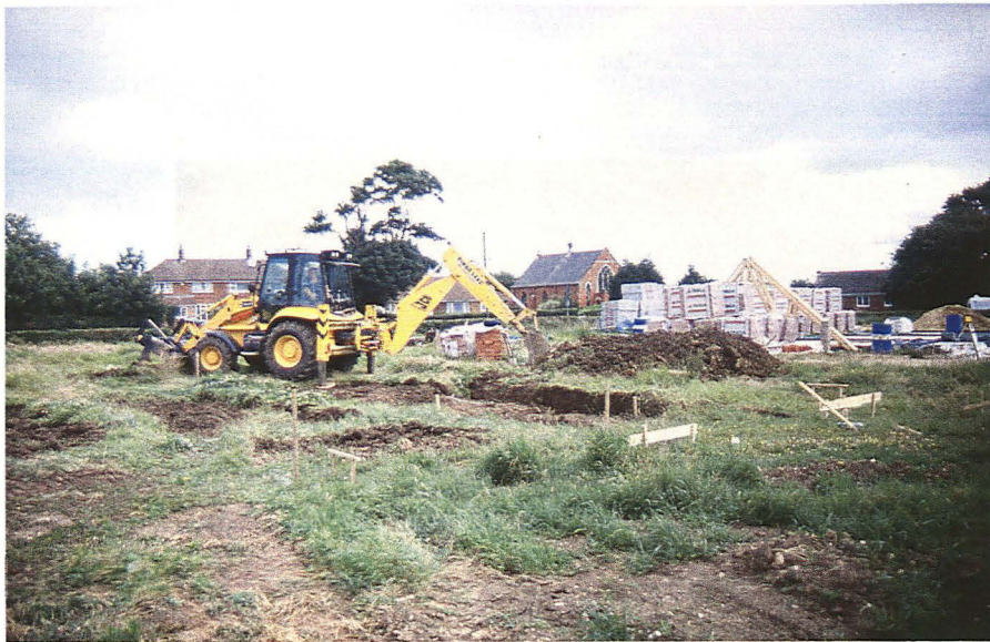
Plate 1 Northeast facing view across Plot 3 during groundworks
