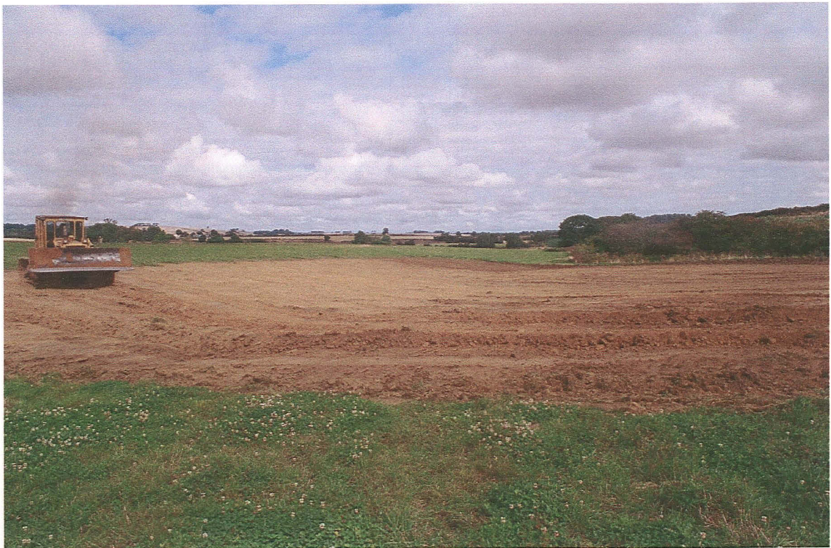
Pl. 2 Natural sands 101 exposed by bulldozer (looking NE).
