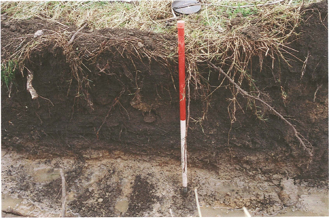
Pl. 3 View of sequence of deposits visible in the west side of service trench (section 2)
