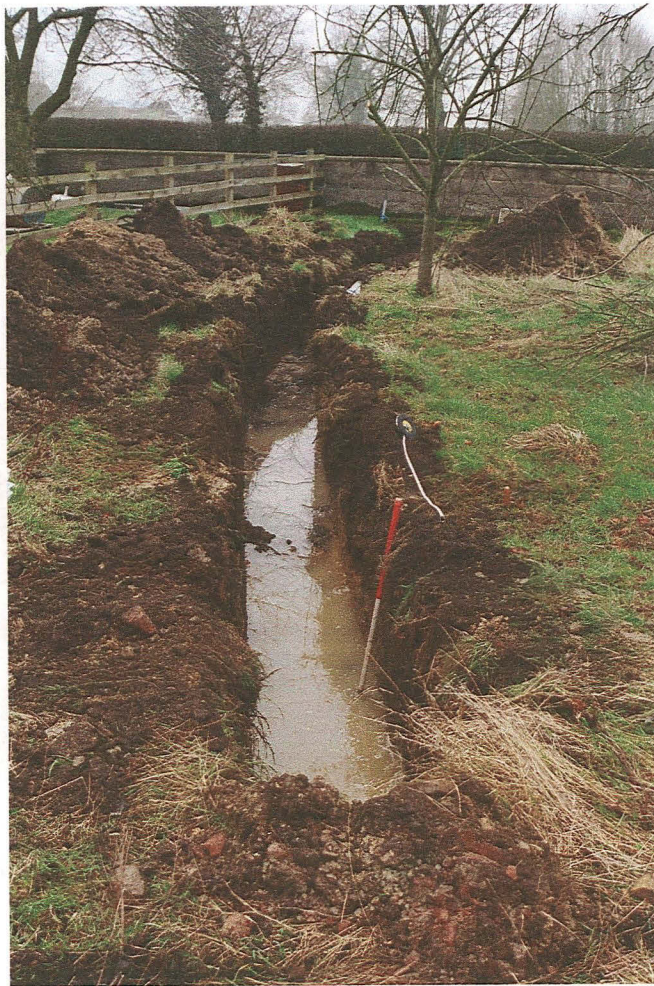
PI. 1 View of the monitored service trench (looking SE)
