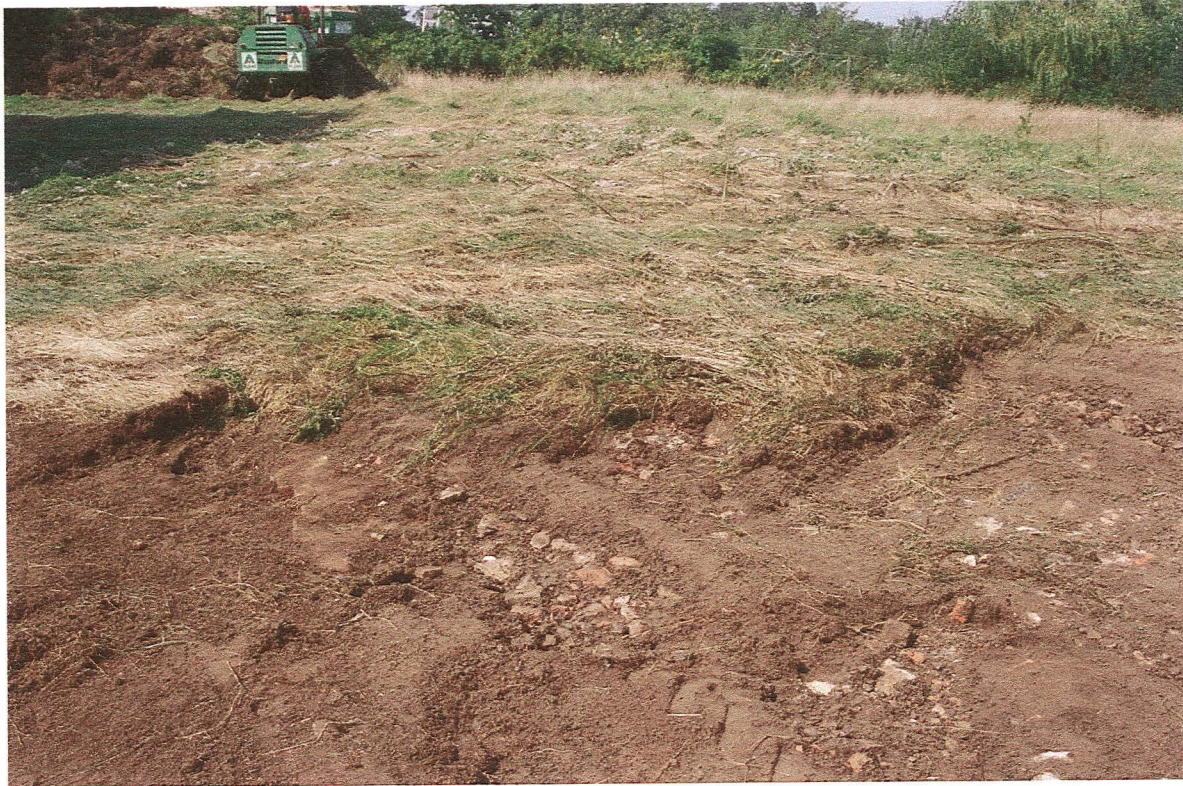
Pl.8 Gravel and brick demolition rubble over the site of a demolished brick structure on the contractors' compound, South Reston (looking NE). The brick wall foundation is in the left foreground.
