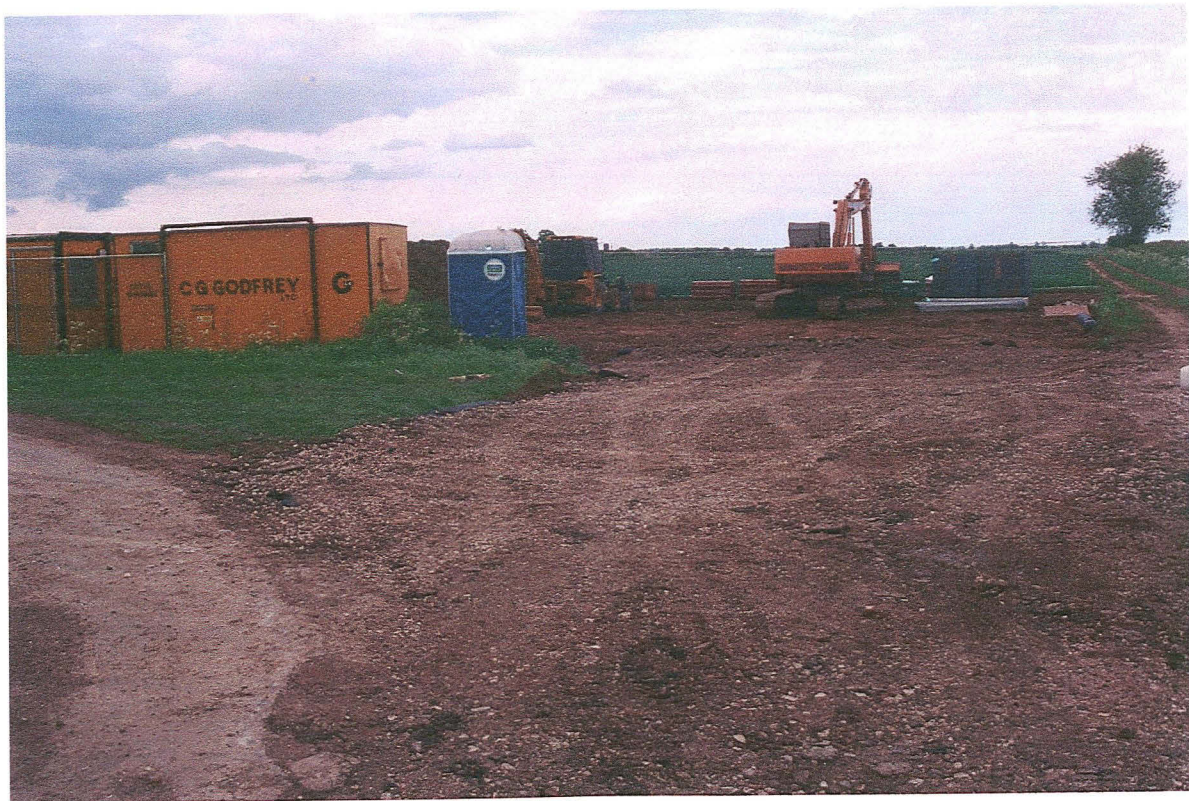
Pl. 4 Contractors' compound site, 32, South Reston (looking east).
