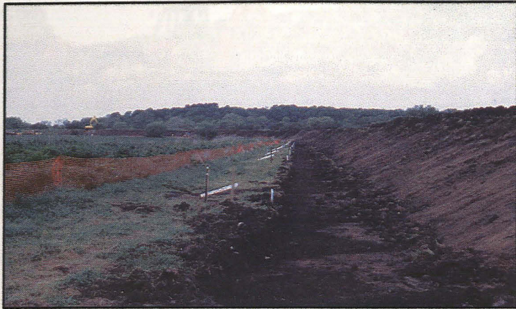
Plate 3: view of section 1, from ch.39820, looking NW.
