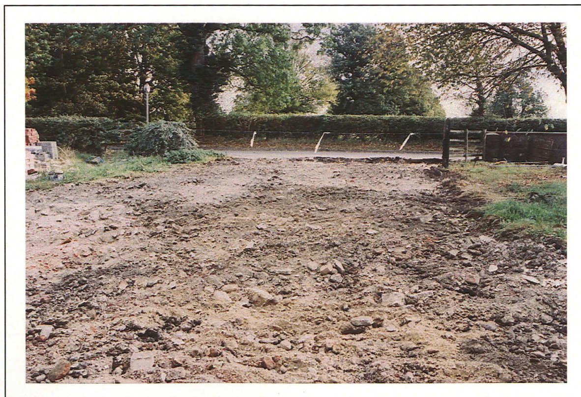
Plate 4: General view of stripped area for new driveway - looking south-east
