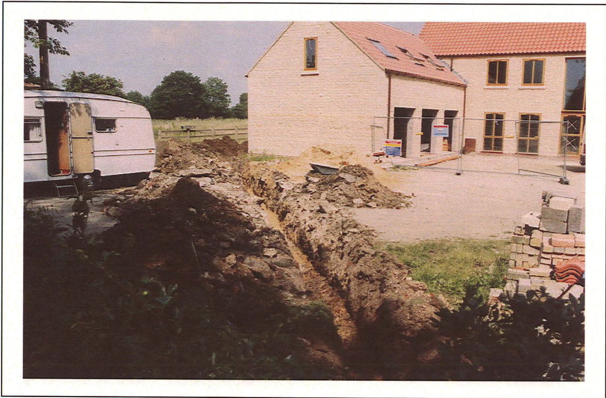
Plate 1: General view of trench for new water main - looking north-west
