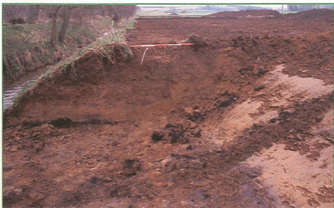
Plate 4 (left): Section cut during excavation of Area 1, looking WSW (upstream).
