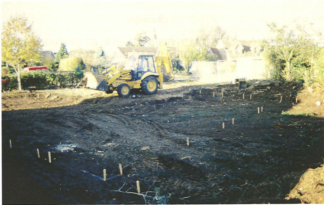
Plate 1 - General view of the development area, looking west
