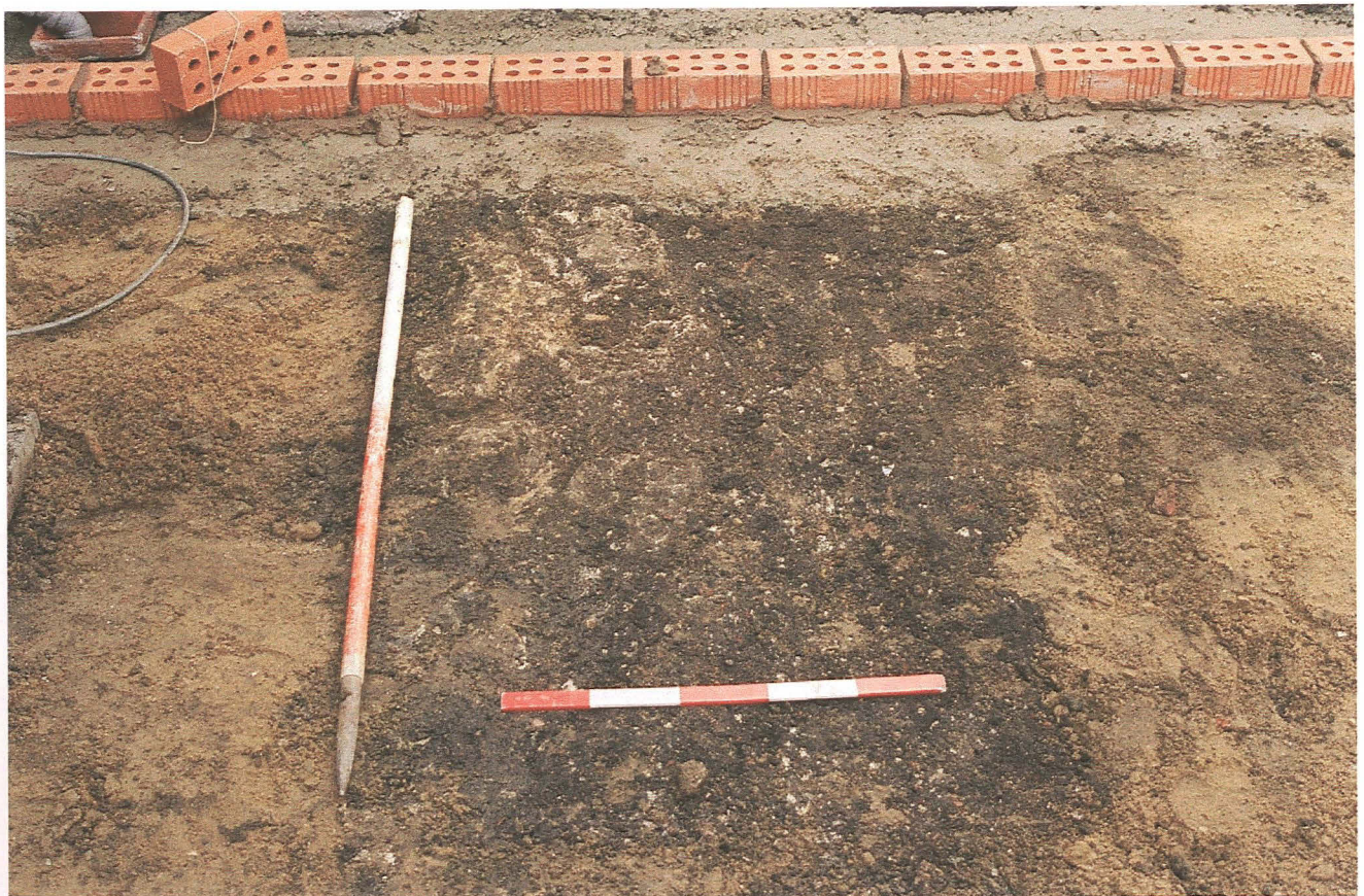
Pl. 8 Wall 3 exposed after the removal of the concrete paving (4) covered by sand bedding (5), looking north. Scales 1m and 0.5m.
