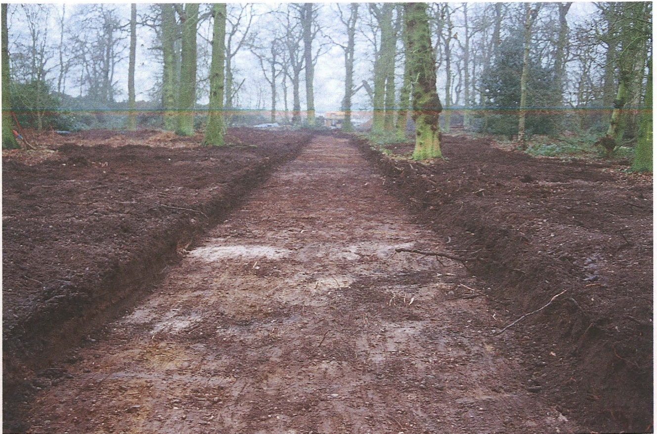
Pl. 18 Path through Tonge's Plantation stripped for the quarry conveyor (looking east).
