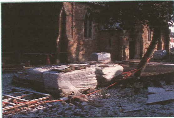
Pl. 2. The churchyard during the enhancement works, looking east.
