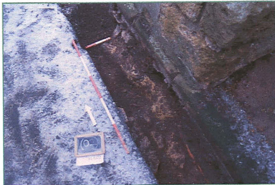
Pl.4. Stone foundation blocks, (002) at the base of the tower buttress, looking north east.
