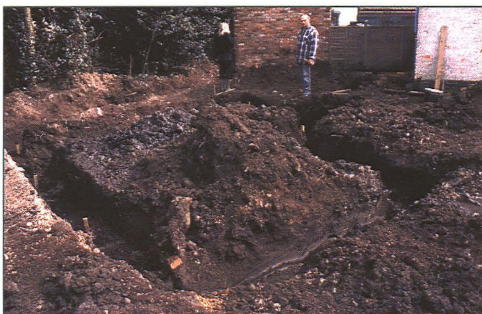
Pl. 2: View of the completed groundworks, looking east-south-east
