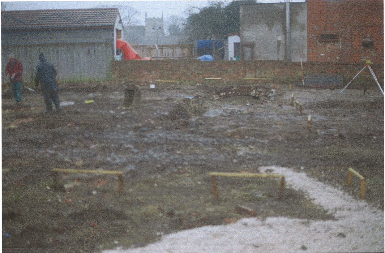
Pl. 1 Plot 2 looking south towards St. Margaret's Church showing the boundary wall.
