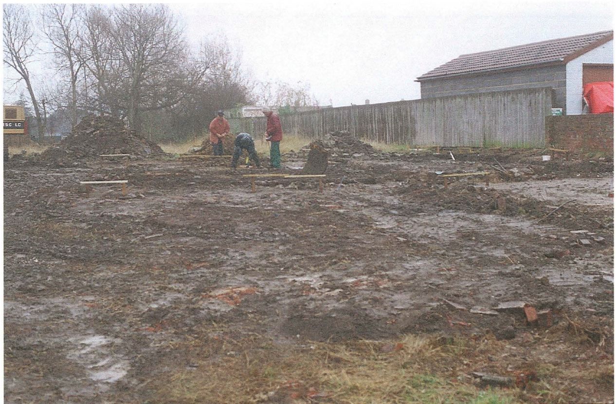
Pl. 2 Plot 2 during excavations with remnants of the brick farm buildings, 105, in the foreground, looking SW.
