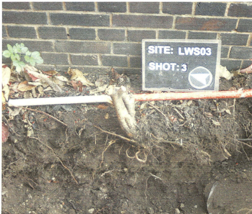
Plate 4 East facing view Section 2, Test Pit 2
