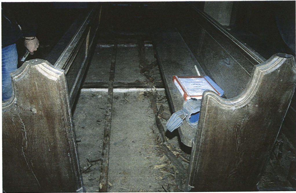
Plate 3 - View showing the exposed timber floor joists and compacted rubble deposit
