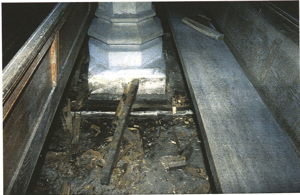
Plate 4 - View showing the exposed base of the nave/south aisle column
