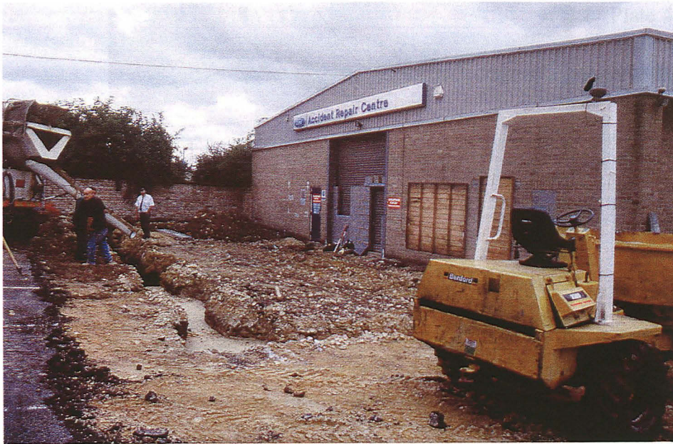
Plate 1 General view, looking east
