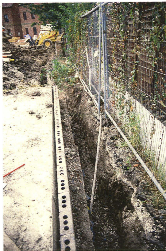
Plate 6 Excavated footings of garage area looking North
