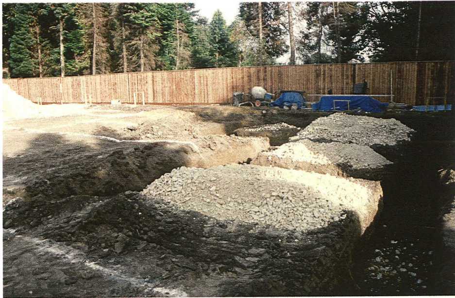
Plate 1 Excavated footings (dwelling)
