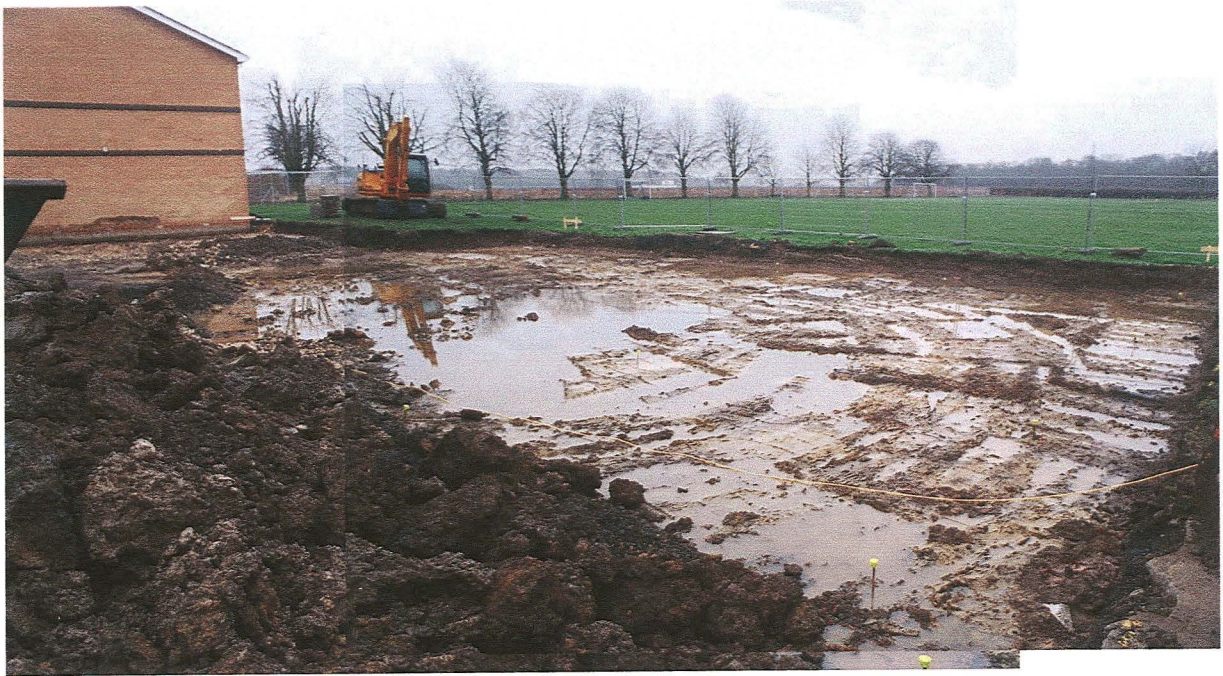
Pl. 1 General view of the site, looking south-west.
