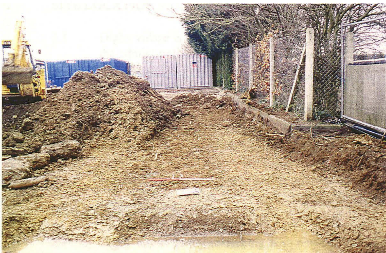
Plate 3 - View of the service trench (007), looking west
