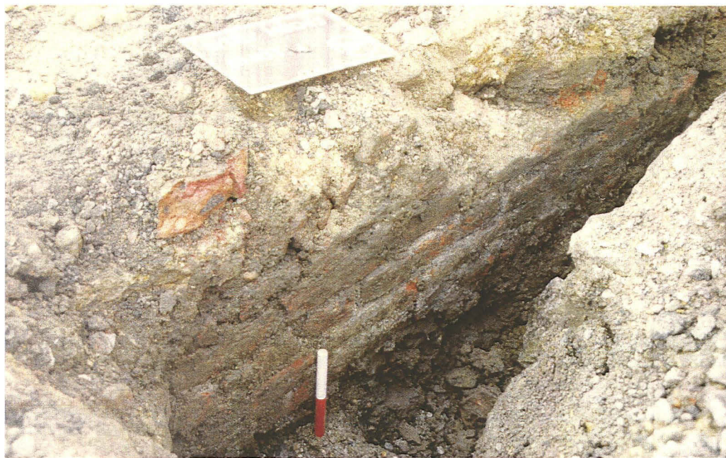
Plate 2 - Section 1 showing wall (002), looking northwest
