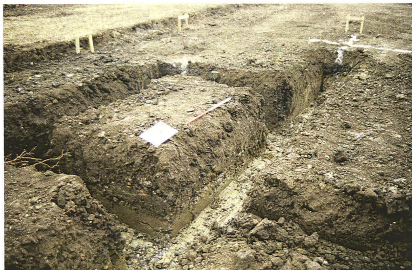
Plate 2 - Section 2 showing Romano-British pit (006), looking southwest
