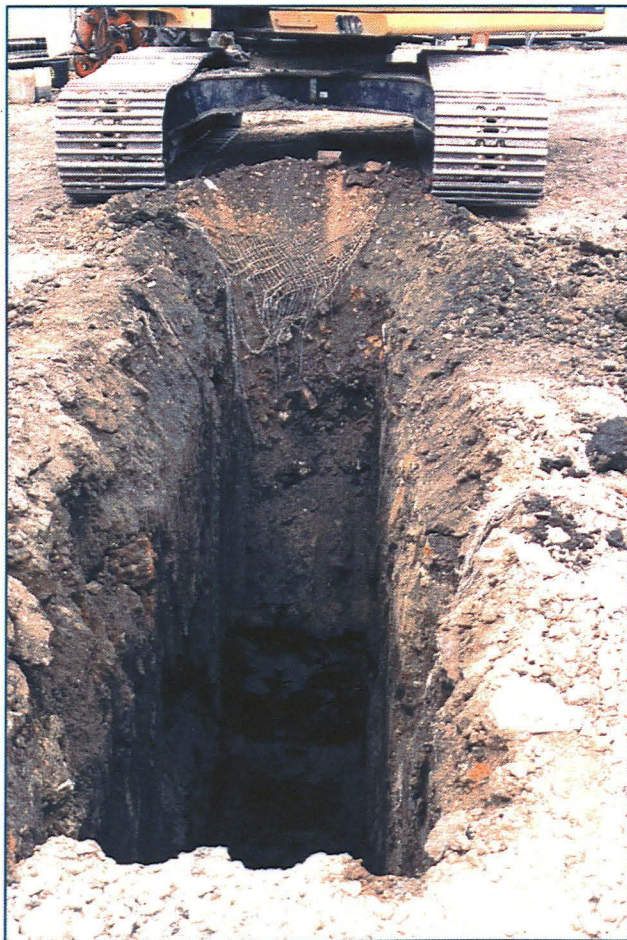
Pl. 2: View of the pit excavated to assess diesel contamination. Looking south-west
