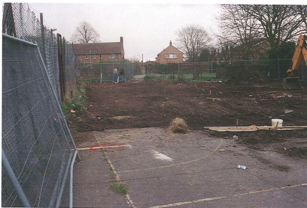
Pl. 1 Position of the monitored four-unit house block (looking east).
