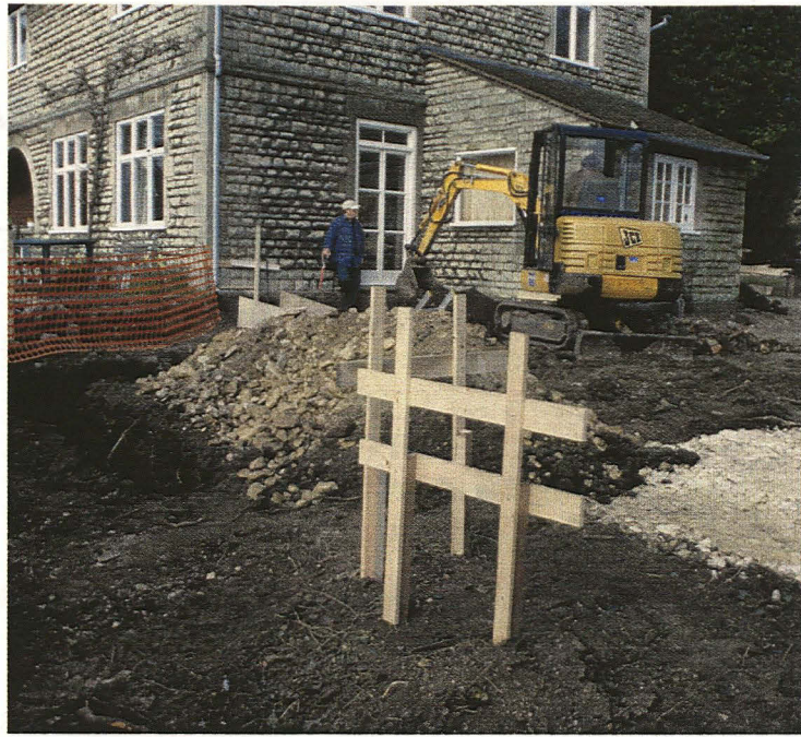
Plate 1 North facing view across groundworks during watching brief
