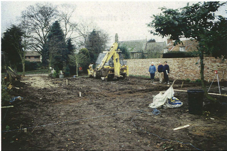
Plate 1 - General view across the site, looking west
