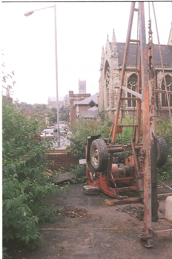
Pl. 8 The augering of Borehole 1.
