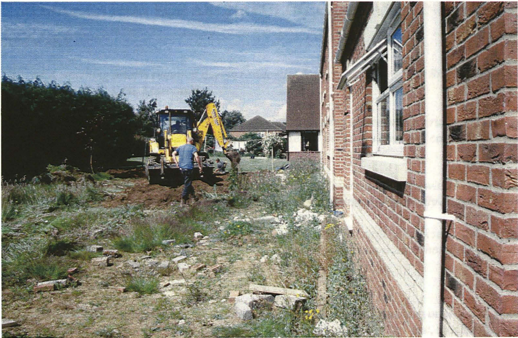
Plate 1 General view of development area showing work being done
