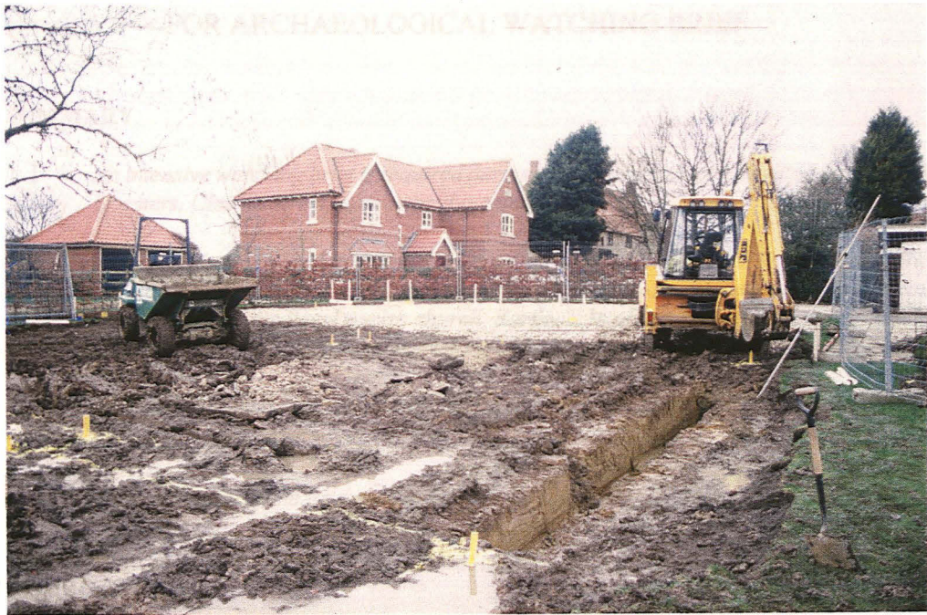
Plate 1 General view of the site during groundworks, looking northwest
