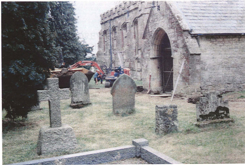
Plate 1 - General view of the drainage works, looking southeast
