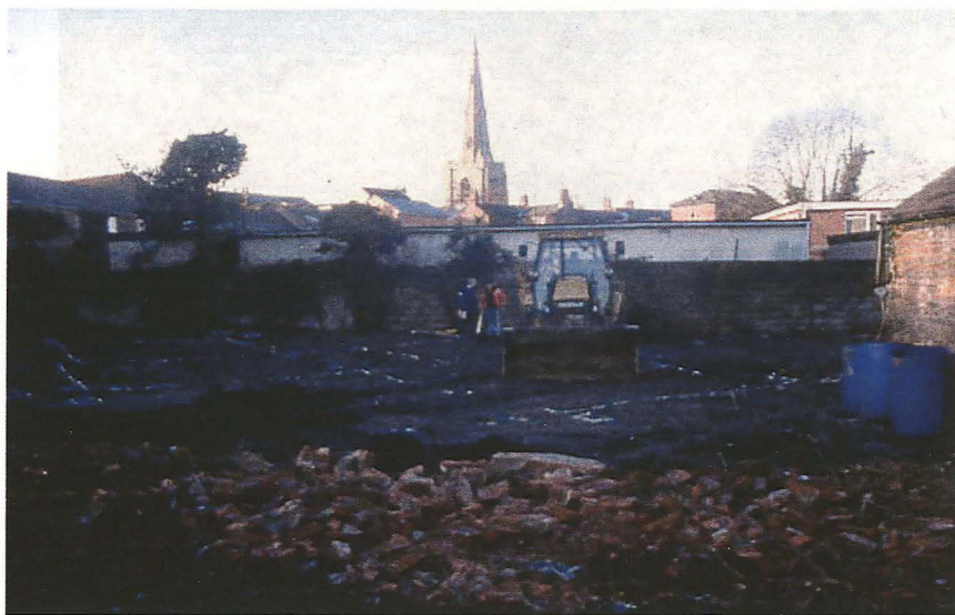
Plate 1 - General view across the development area, looking southwest
