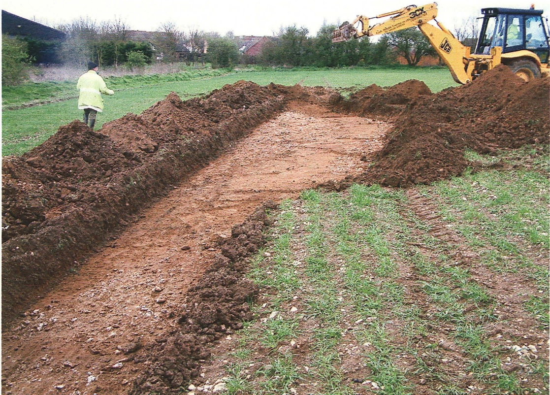
Plate 8. Trench 5 after extending showing linear feature.
