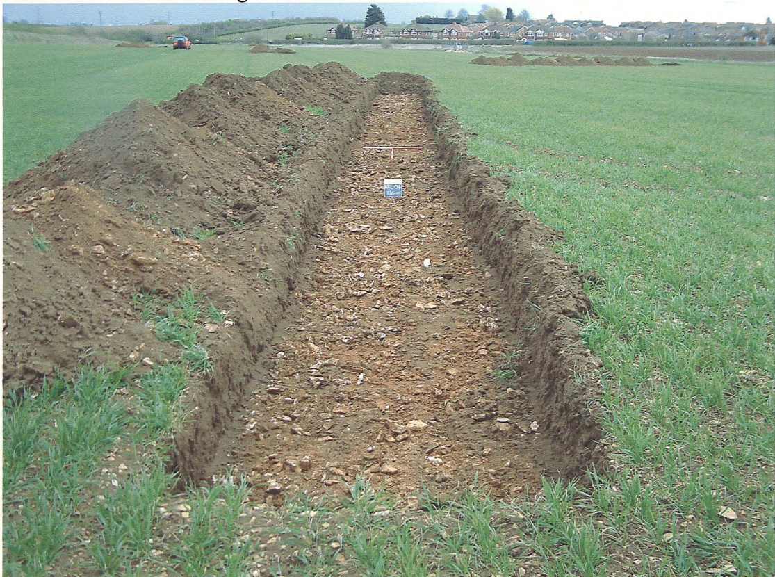
Plate 24. Trench 14 looking south east.
