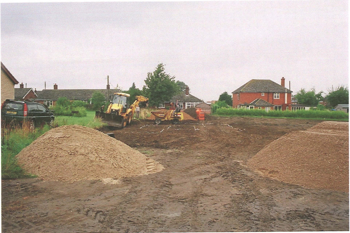
PI. 1 Plot 1, prior to excavation of the foundation trenches. The plot had been raised with redeposited material and the development site had been stripped of topsoil (looking north to Pinnings Lane).
