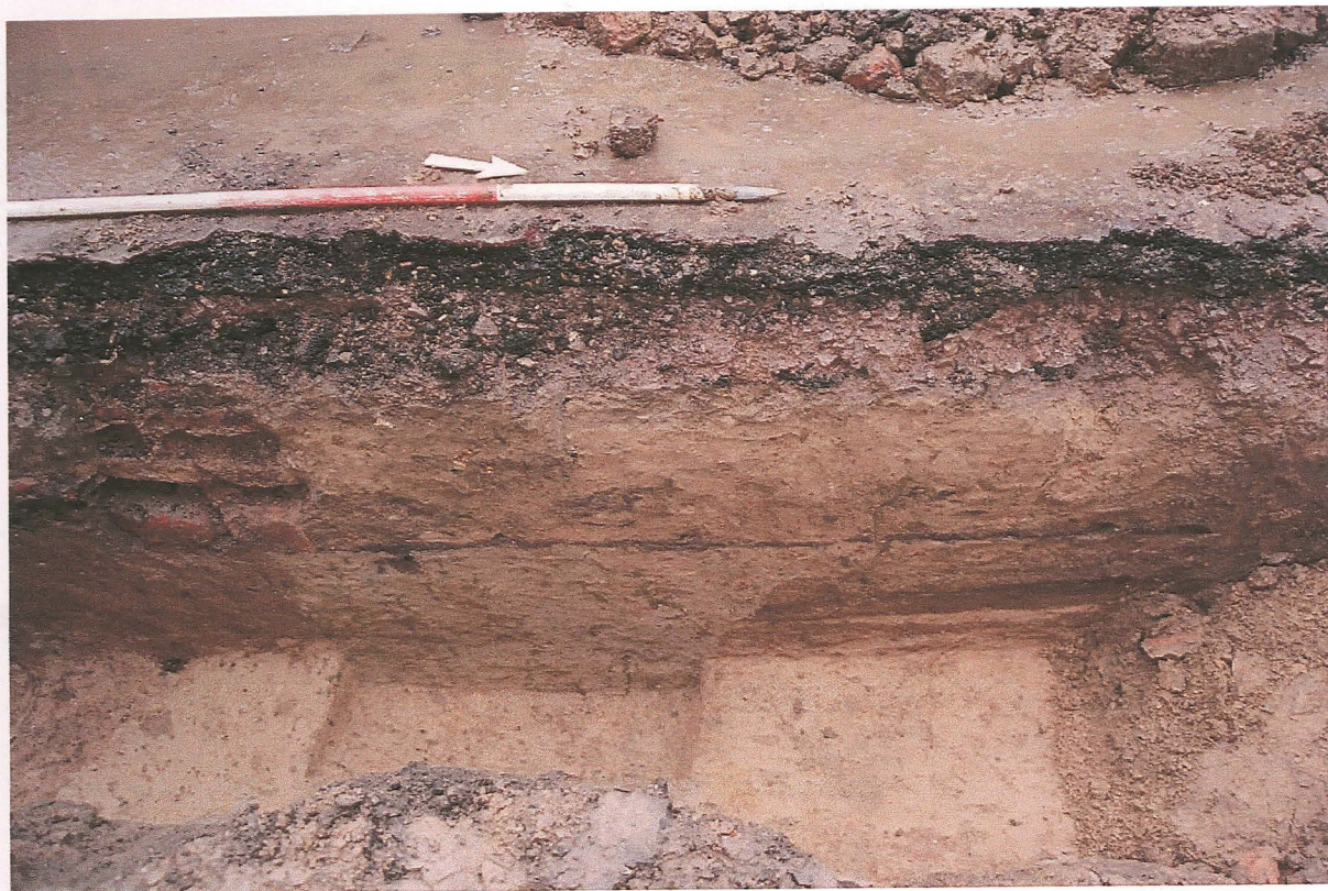
Pl. 6 Western foundation showing brick wall 109, ditch 115 and occupation layer 130, looking west. Scale 2m.
