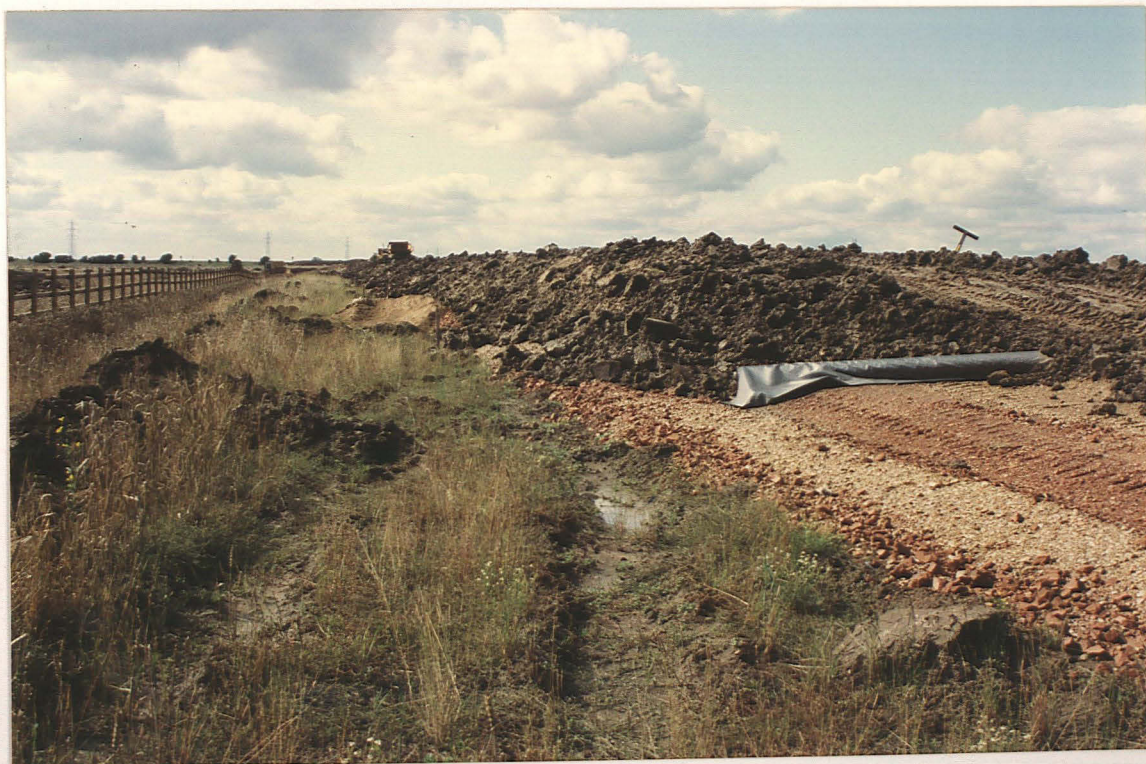
Pl. 28 The borrowpit was used to supply clay for consolidating the brick rubble base of the A16 Spalding Bypass.
