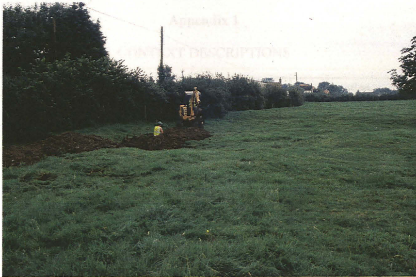
Plate 1 - View showing the cable trench during excavation, looking west
