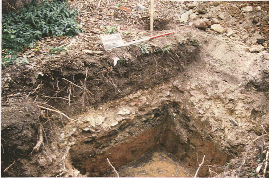
Plate 14. Southeast facing view of Soakaway 1 prior to cleaning.
