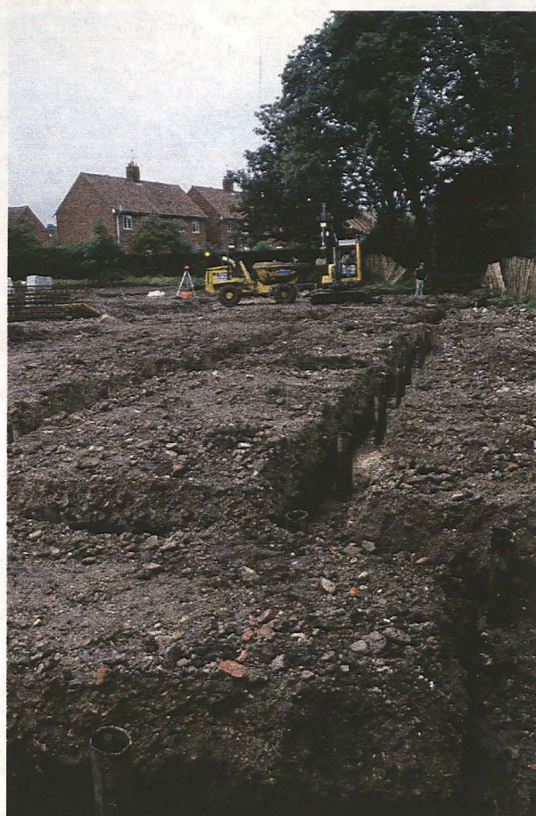
Plate 2. East facing view showing groundworks being undertaken for Block C.
