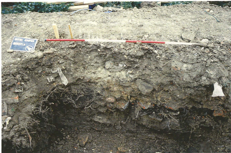
Plate 3 Section 1, looking northeast
