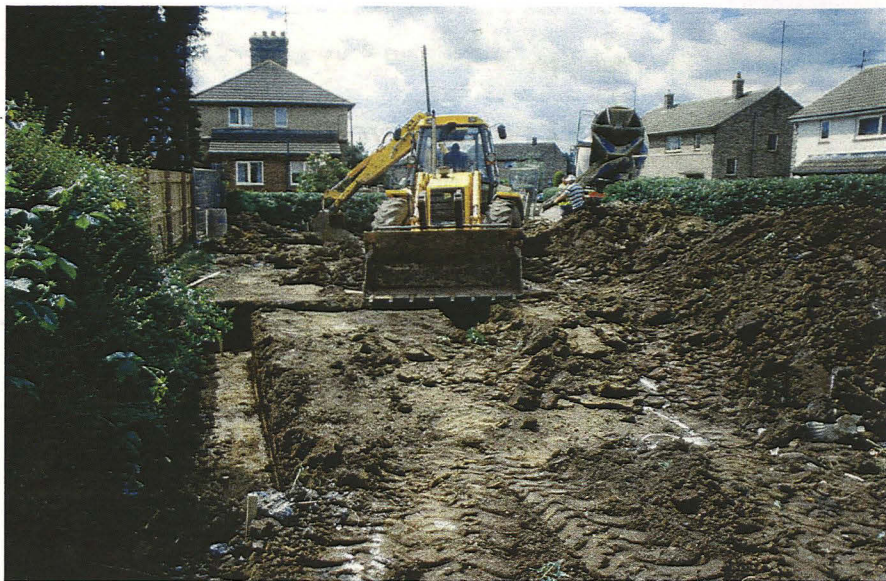
Plate 1 - General view across the development area, looking southwest
