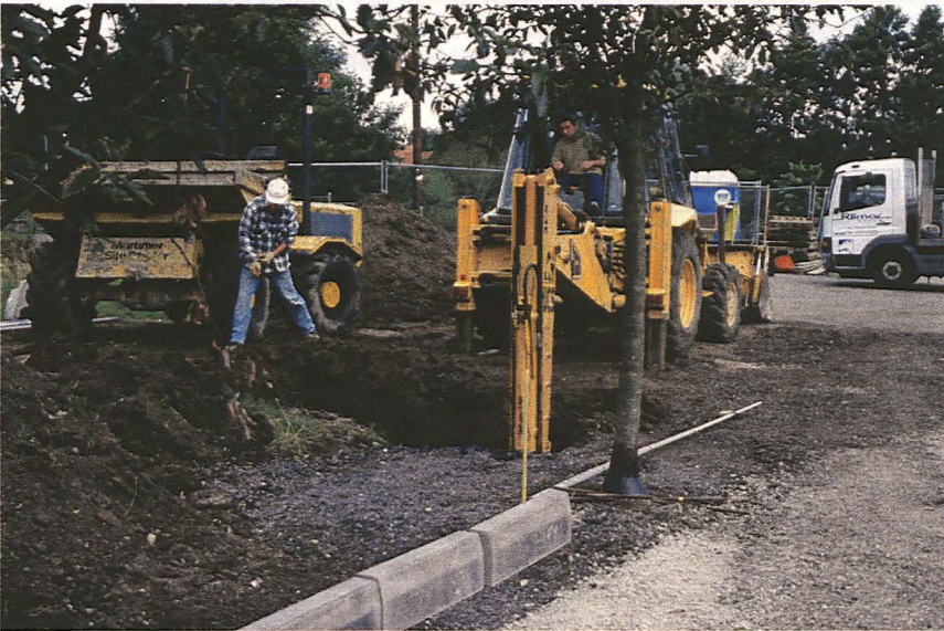
Plate 2 - Excavation of the Interceptor Pit in progress, looking west
