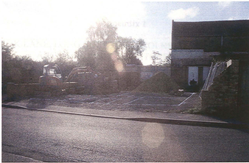
Plate 1 - General view across the development area, looking southeast
