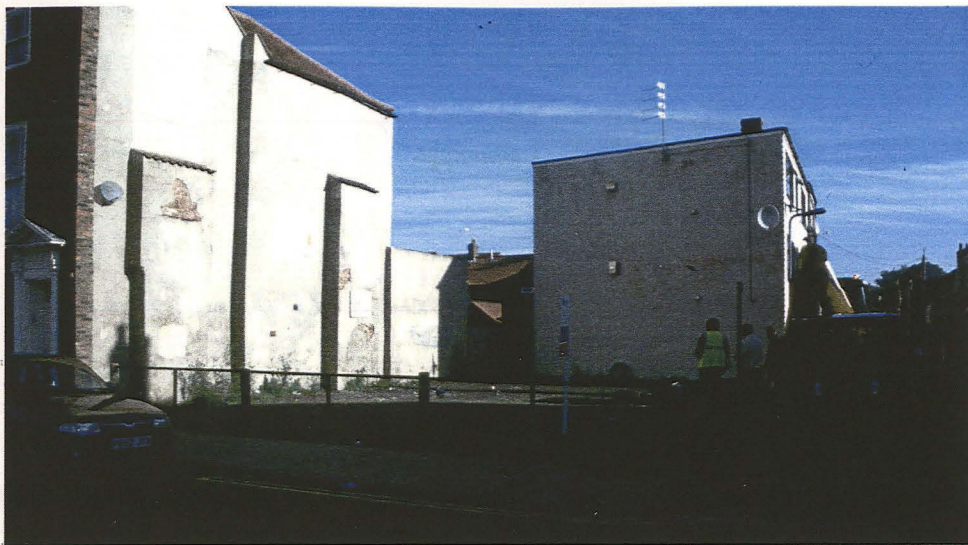
Plate 1 General view of site, looking northeast
